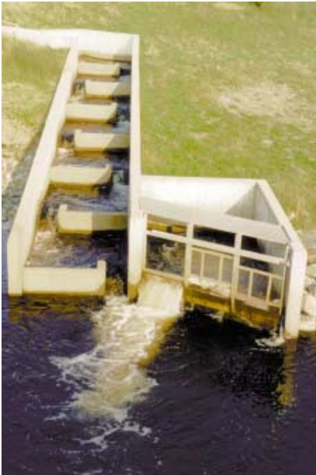
Fishway, Ruth Falls dam, East River Sheet Harbour, N.S.
