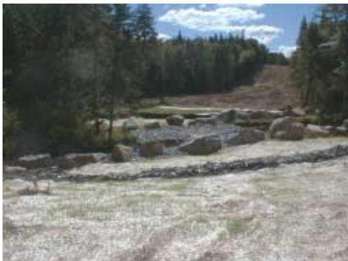
Pipeline crossing with proper sediment and erosion control for the protection of fish habitat.
