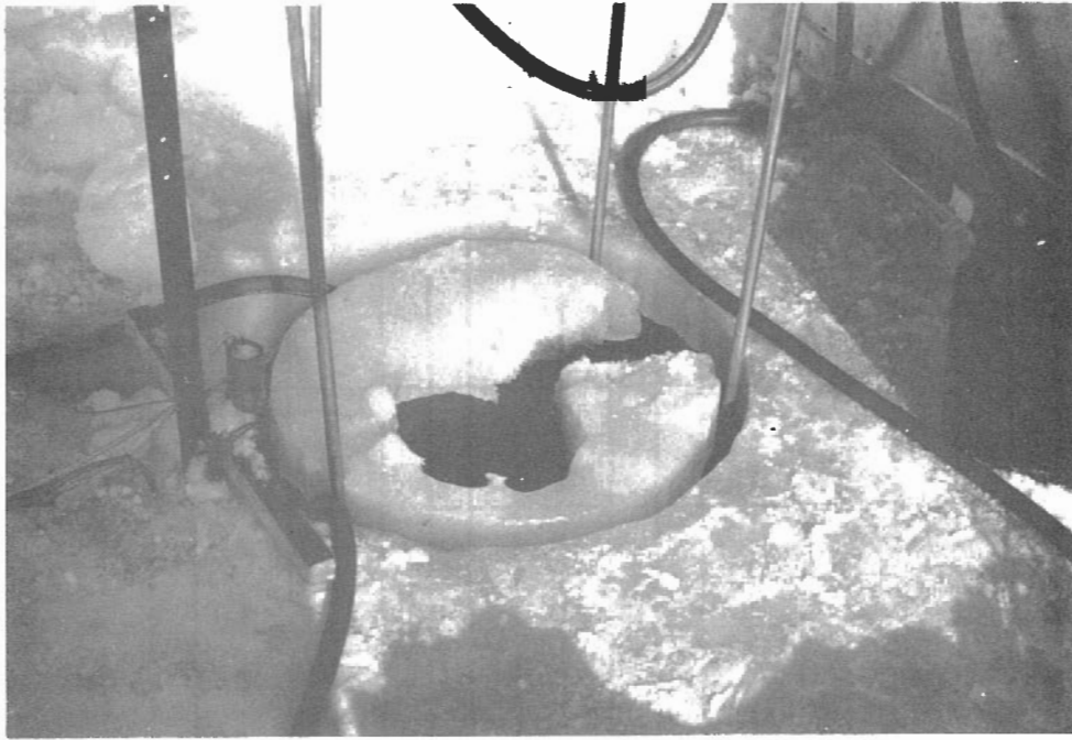
Closeup of Ice Melting Equipment
