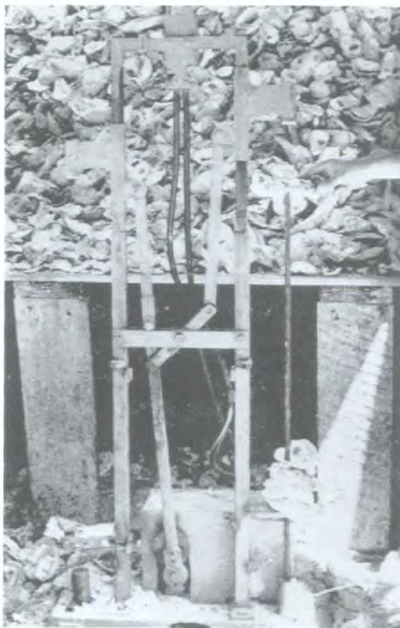
FIG. 55. Machine for punching oyster-shell culch.
